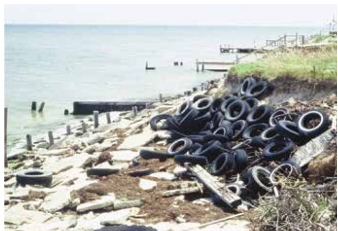
A landowner has attempted to resolve shoreline erosion by piling tires and debris, a method that will not work long-term.
